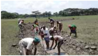
Excavating field channel in polder the 43/2A
