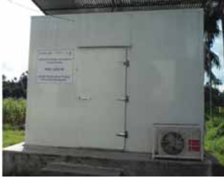
Fig 14: CoolBot storage system
