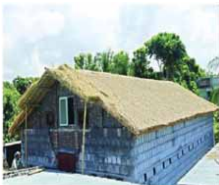
Fig 11: Natural store of 300 MT capacities using the technology of evaporation
